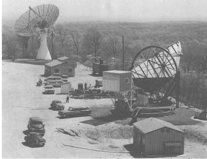
Figure 9: The 20-foot “home-made” horn reflector antenna in the foreground designed by A. B. Crawford (head of the Bell Labs department I joined in 1961) served as the Lab’s receiving station for Echo, the world’s first communications satellite project. Unlike this horn antenna, whose response pattern is tightly grouped about its main beam, the commercial 60-foot (diameter) parabolic antenna, shown in the background, picks up an appreciable amount of radiation from the ground, via spillover of the (downward-facing) feed horn located at its focus.
